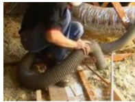
Insulation Removal
